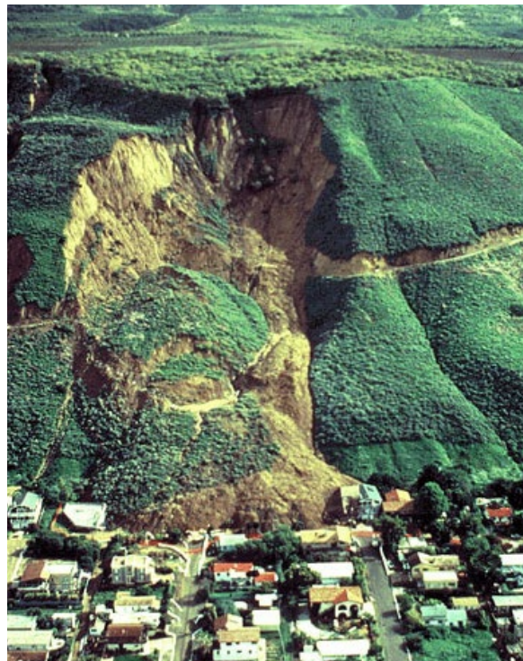
1995 La Conchita, CA landslide
